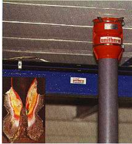
Palusol based in tumescent plastic pipe device used for commercial fire stopping.
