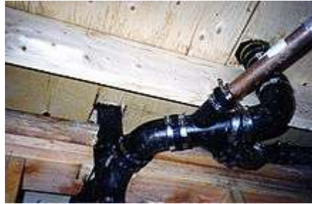
Cast iron drain, waste and vent piping
