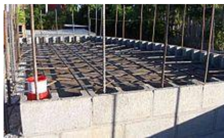
Suspended slab formwork and rebar in place, ready for concrete pour. On reinforced concrete block work supporting walls.
