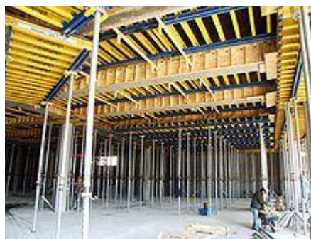
Form work tables in use at a building site with more complicated structural features
