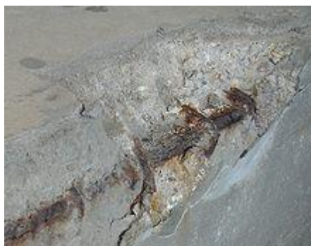
Concrete spalling caused by the corrosion of rebar Main article: Concrete degradation
