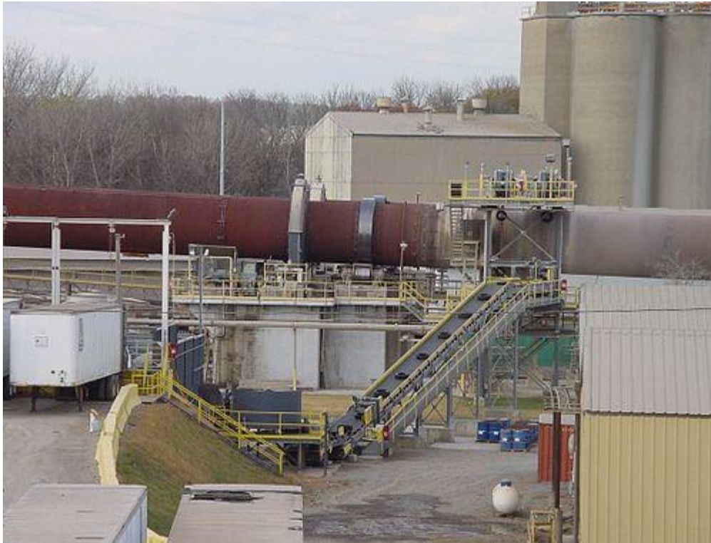
Used tires being fed mid - kiln to a pair of long kilns
