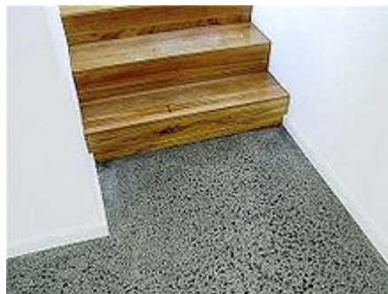
New polished concrete floor
