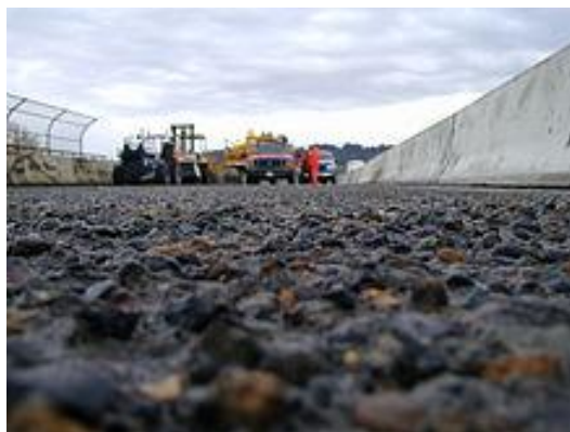
Exposed clean aggregate left by scarification
