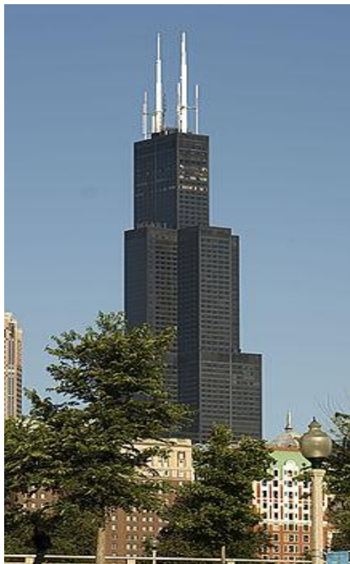
The Willis Tower showing the bundled tube frame design
