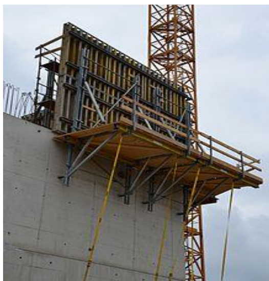
Crane - Climbing formwork : The working platform and the formwork are a unit
