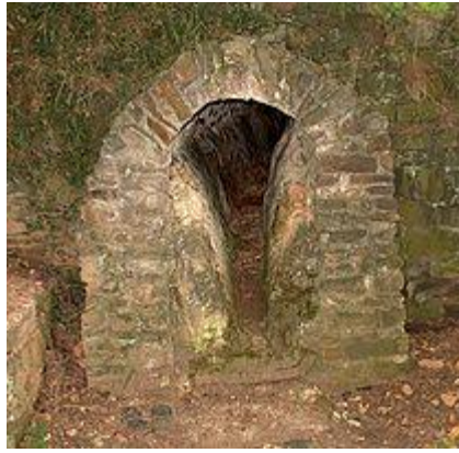
A portion of the Eifel aqueduct , Germany, built in AD 80, showing the calcium carbonate that accretes on the sides of the channel without regular maintenance
