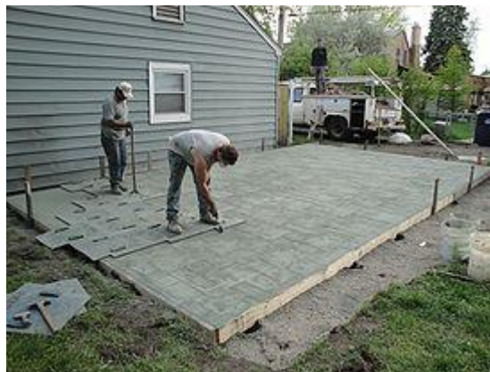
Concrete being stamped with an Ashlar Slate pattern
