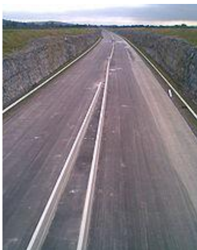
The concrete step barrier in the under construction M8 motor way in Ireland ( August 2008 ) .
