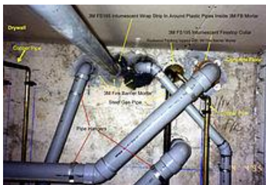
Plastic pipes penetrating a concrete floor in a Canadian highrise apartment building
