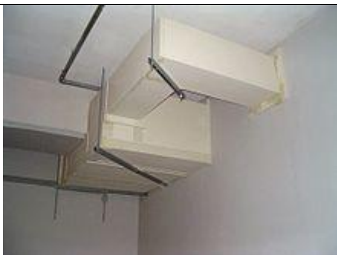
Circuit integrity fireproofing of cable trays, using calcium silicate boards.
