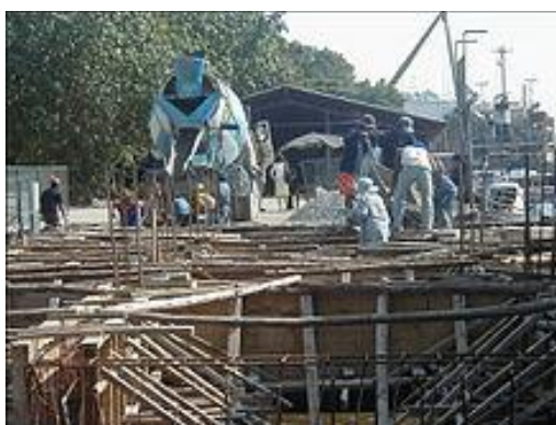
Traditional timber Form work on a jetty in Bangkok
