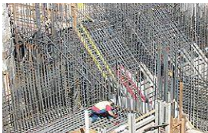
Rebar for foundations and walls of sewage pump station.
