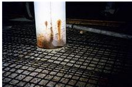
Hydro demolition around column
