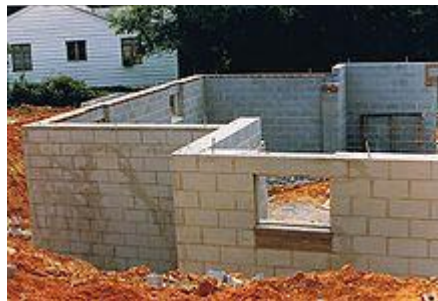
Concrete masonry units (CMUs) or blocks in a basement wall before burial.
