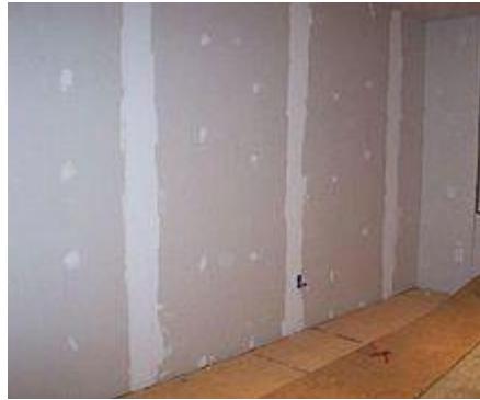
Vertically hung drywall with joint compound.
