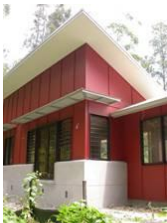
CSR Fiber Cement sheet cladding - dwelling addition, Hardys Bay, NSW, Australia
