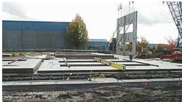
A tilt-up building during construction. A cast wall section is being righted. Other sections are visible in their forms .
