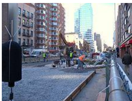
Crushed stone being laid to underlie a road surface
