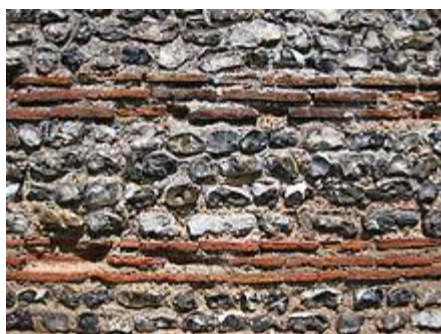
Detail of the wall of the Roman shore fort at Burgh Castle , Norfolk, showing alternating courses of flint and brick work.
