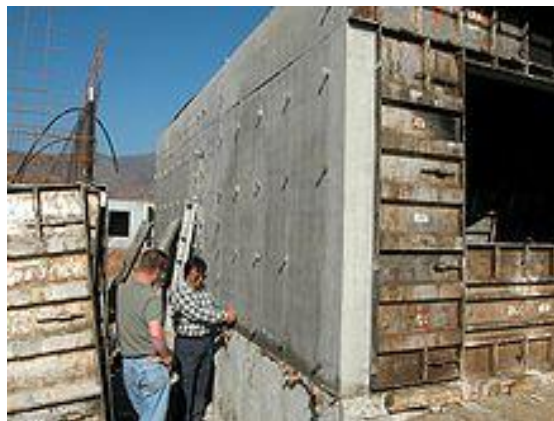
Form work stripped exposing the set concrete
