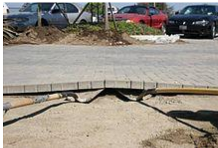
Pavers Being lifted to demonstrate interlock
