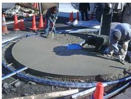
Pouring and smoothing out concrete at Palisades Park in Washington
