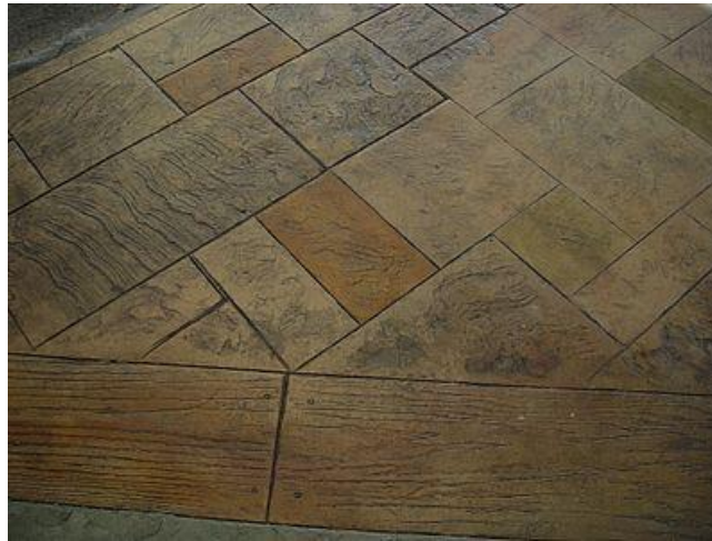
Stamped Concrete in various patterns , highlighted with acid stain )
