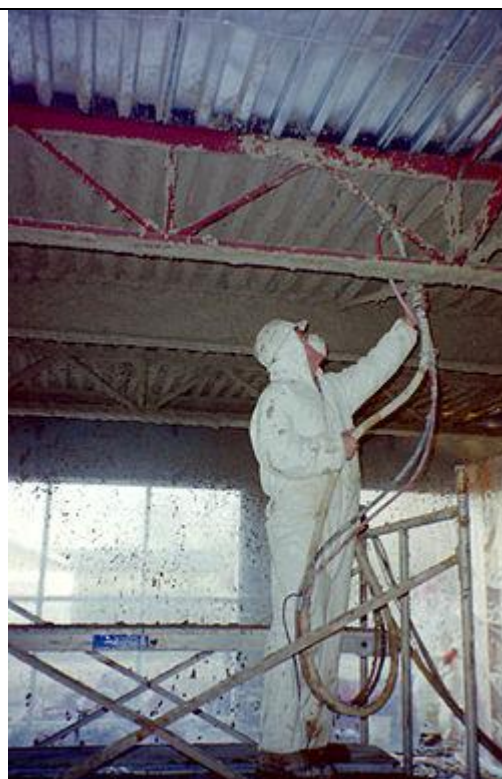
Spray gypsum based plaster fireproofing being installed.
