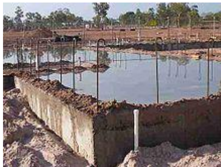
A concrete slab pounded while curing.
