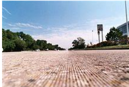
Results of diamond grinding of pavement
