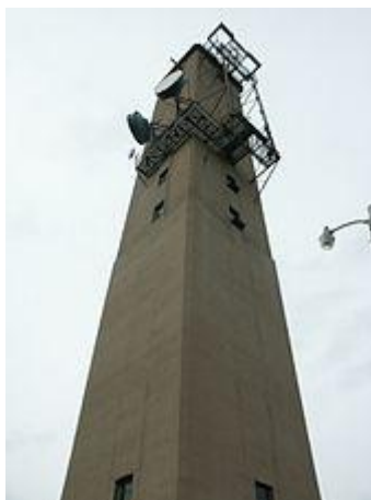
AT&T Long Lines relay tower in Indiana constructed with the slip - form method.
