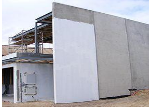
A precast concrete walled house in construction
