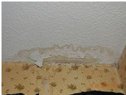
Drywall water damage in a closet.
