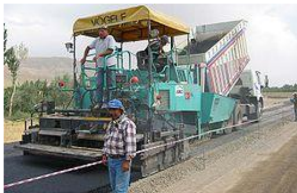
Machine laying asphalt concrete, fed from a dump truck.
