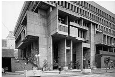
A modern building: Boston City Hall (completed 1968) is constructed largely of concrete, both precast and poured in place.
