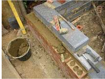
Laying bricks with portland cement mortar
