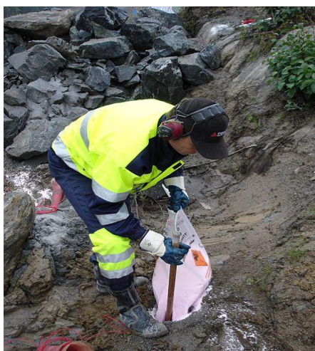
Charging a hole with ANFO for rock blasting
