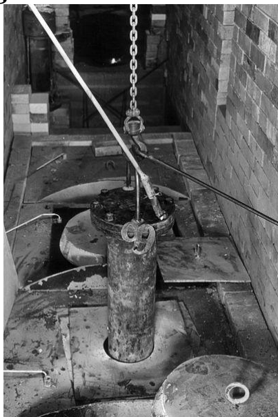
A "bomb" (pressure vessel) containing uranium halide and sacrificial metal, probably magnesium, being lowered into a furnace
