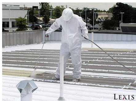
Coating on a roof
