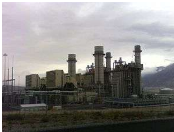
Currant Creek Power Plant near Mona, Utah is a natural gas fired electrical plant.
