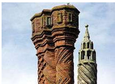
Carved brick chimneys characteristic of late Gothic Tudor buildings, at Thornbury Castle, 1514
