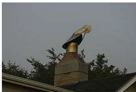
Spanish Conquistador style wind directional cowl found on many homes along the windy Oregon coast.
