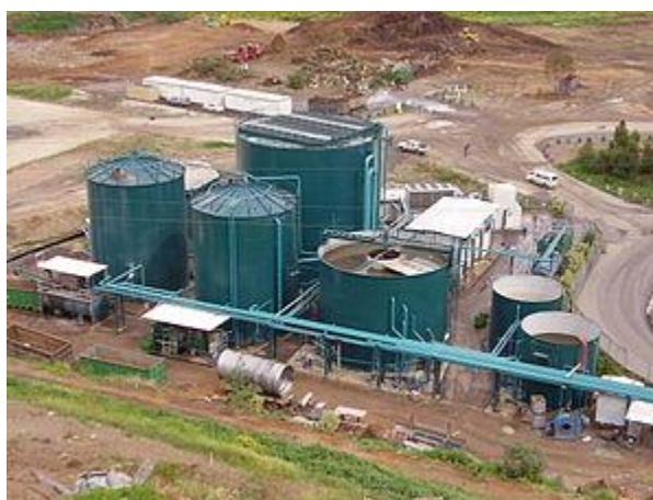
Two-stage, low solids, UASB digestion component of a mechanical biological treatment system
