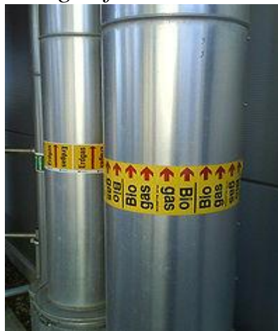
Biogas carrying pipes
