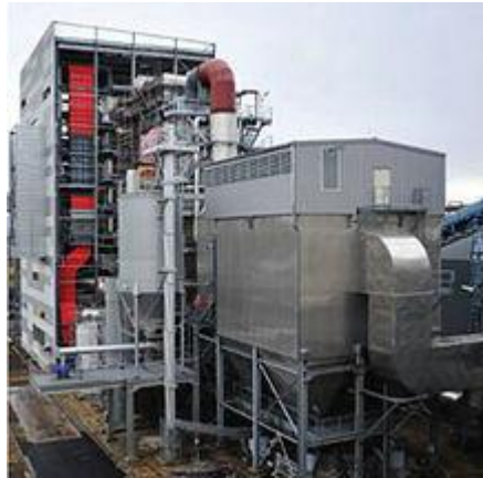
A cogeneration station in Metz, France. The 45MW boiler uses waste wood biomass as energy source.
