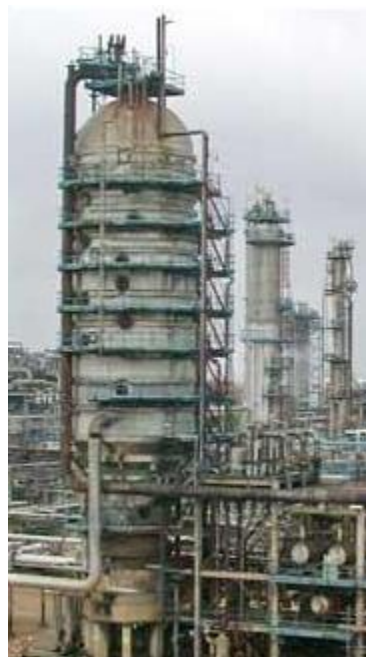
Large - scale, industrial vacuum distillation column
